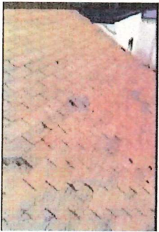
top of Roof 2 .png 850K
